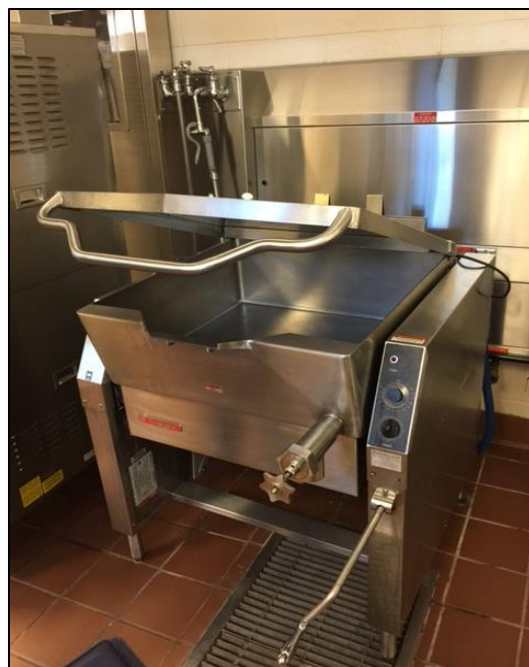
Tilt skillet with broken temperature dials at Luke C. Moore.
