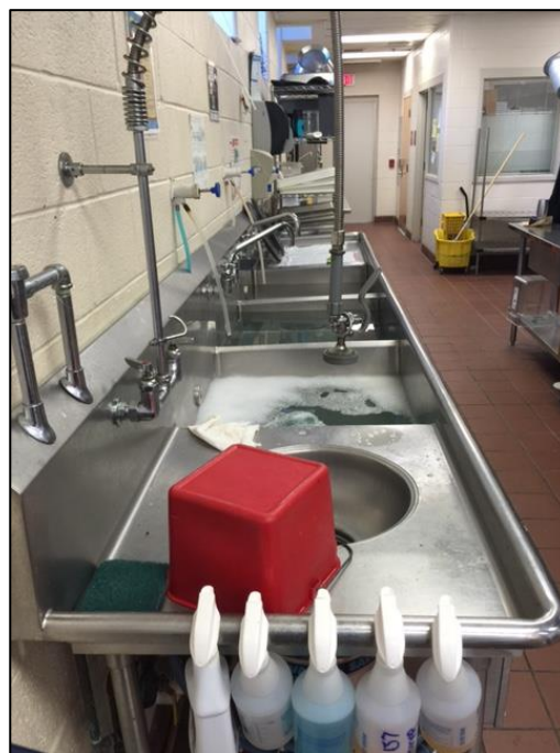
Sink with broken garbage disposal at Luke C. Moore.
