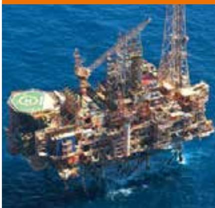
Located off the north-west coast of Australia, the Western Flank B project develops five fields via an eight subsea well tieback to the Goodwyn A platform.
